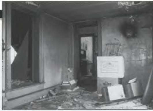
AEBM Caretaker Suite BEFORE renovation.
